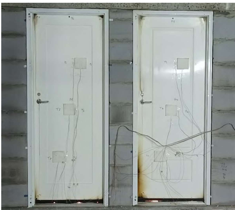
Fig. 4 Unexposed Side after 20 Minutes
